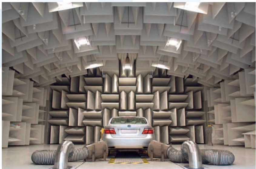
The same site, once the chamber was completed and the wedges installed
