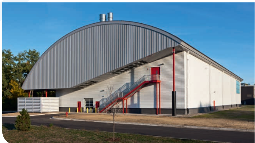
Typical building shape from outside a turnkey facility with a curved roof
